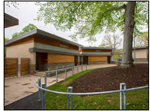
New Restrooms at Merriweather Post Pavilion
