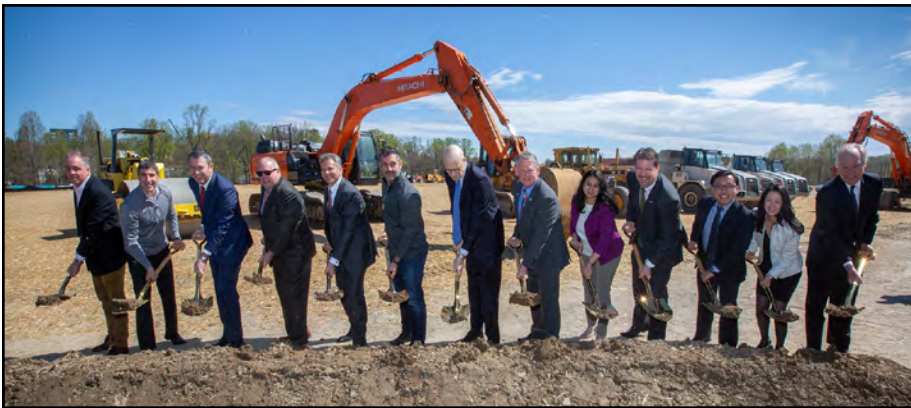
Groundbreaking for Area 3 of the Crescent Neighborhood included Maryland Governor Larry Hogan, County Executive Allan H. Kittleman, members of the Howard County delegation, and other elected officials and business leaders.
