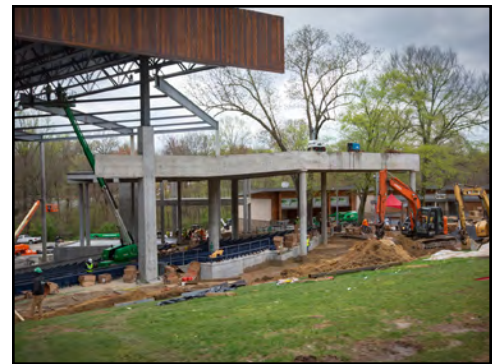
Merriweather under renovation in 2018
