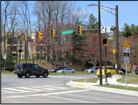
Improved intersection of Hickory Ridge Road and Broken Land Parkway
