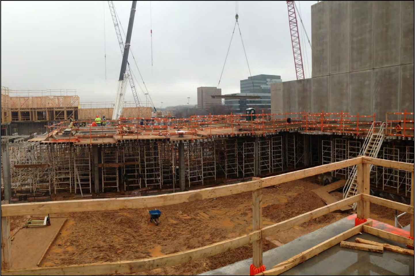
The Metropolitan under construction in Warfield
