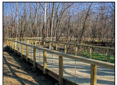
The new Lake Kittamaqundi Loop pathway crosses a wetland on an elevated boardwalk.
