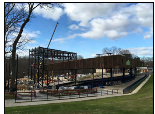
Renovations at Merriweather Post Pavilion
