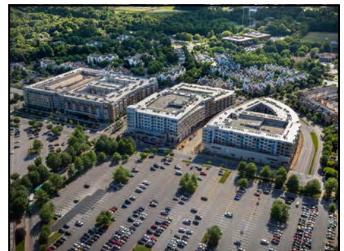
The Metropolitan (left), TEN.M (center), and m.flats (right)
